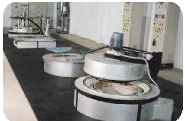
Heat Treatment Plant
